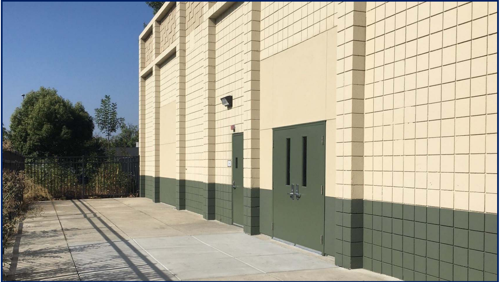
Morrill – Music Room HVAC Upgrade Exterior
